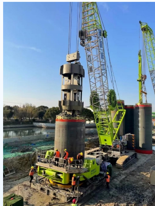
Bored Pile Construction
