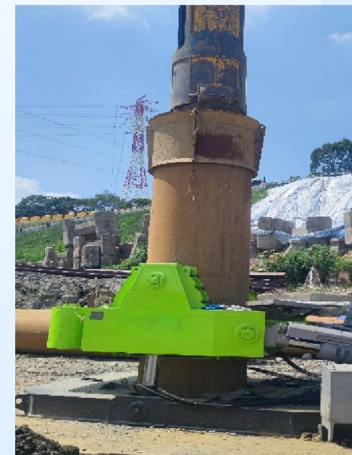
River Bank Drilling Construction
