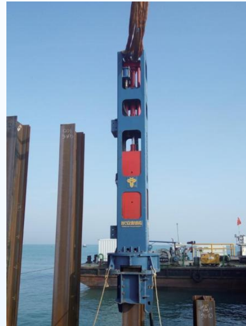
Israeli Port Construction Site
