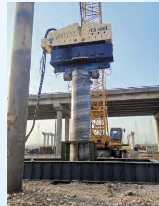
Light Rail Project
