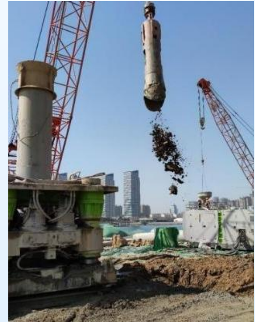
Subway Station Construction
