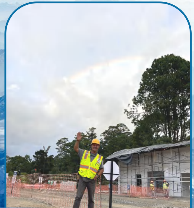
Project location: Guatemala Product: Steel Plate, Steel pipes Steel Consumption: 2200 tons Application: Church construction
