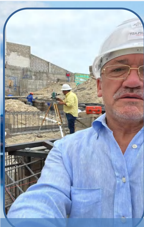
Project location: Ecuador Product: Steel Plate&Rebar Steel Consumption: 3200 tons Application: Warehouse construction
